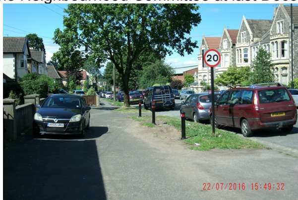
Westbury Road Bollard Installation
