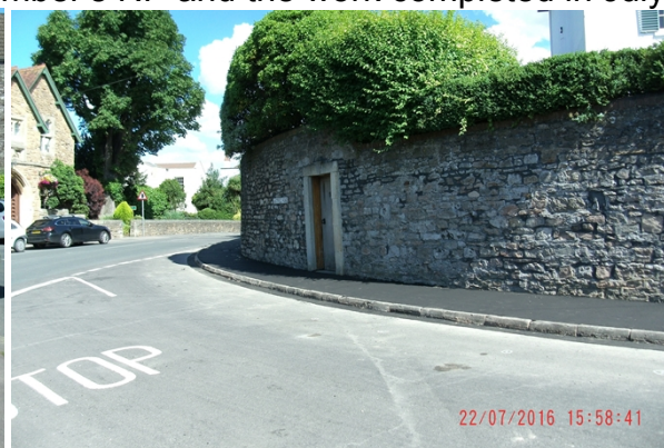
Eastfield Road Pavement Realignment
